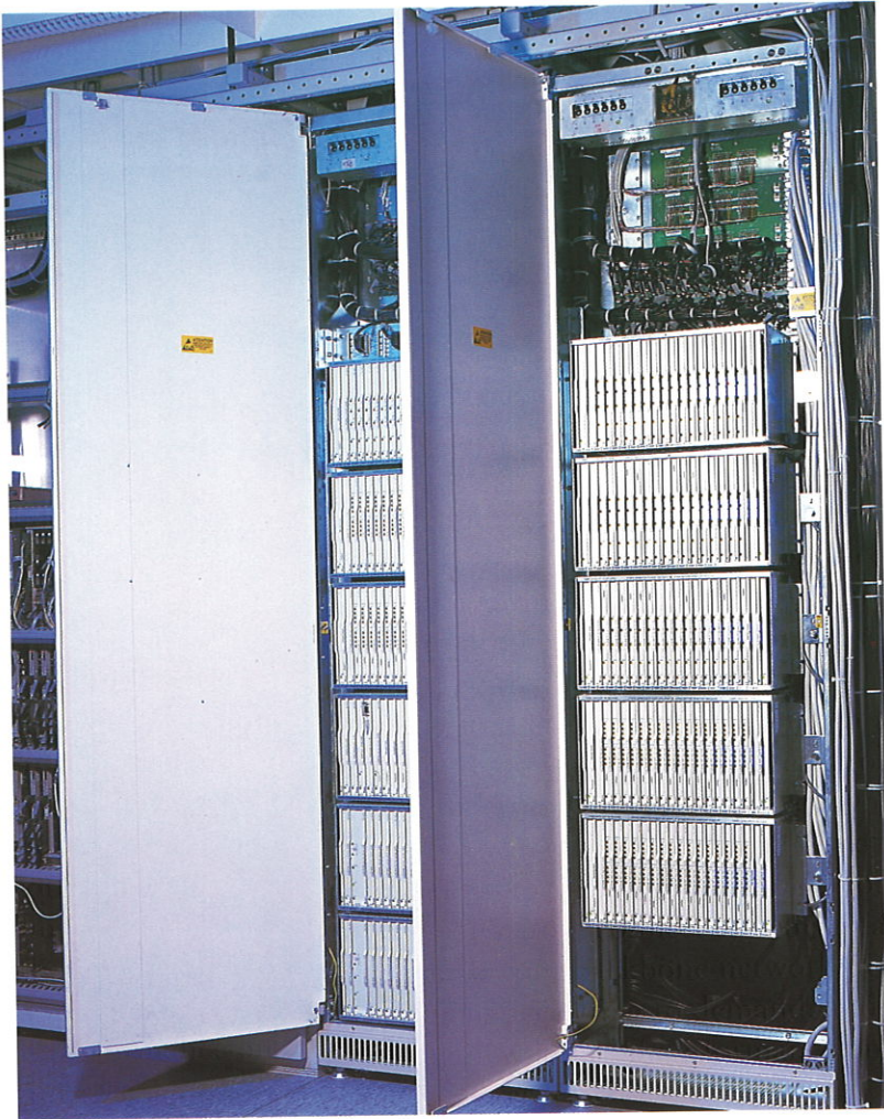
With systems like Ericsson's cross-connects, you can bring configuration flexibility to PDH transmission networks.
