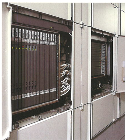
The AXD 4/1 system switches and cross-connects 2, 34 and 140 Mbit/s PDH systems, and provides a 'bridge' from PDH to SDH transmission.
